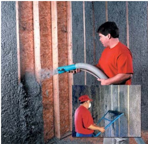
Applegate cellulose being sprayed into a new home
