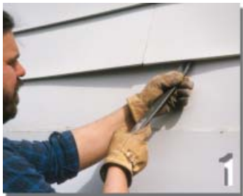
Siding is carefully removed
