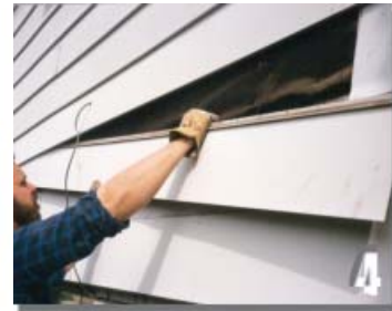
Siding is replaced
