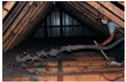
Installing Applegate Stabilized™ insulation
