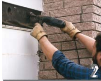
Small holes are drilled
